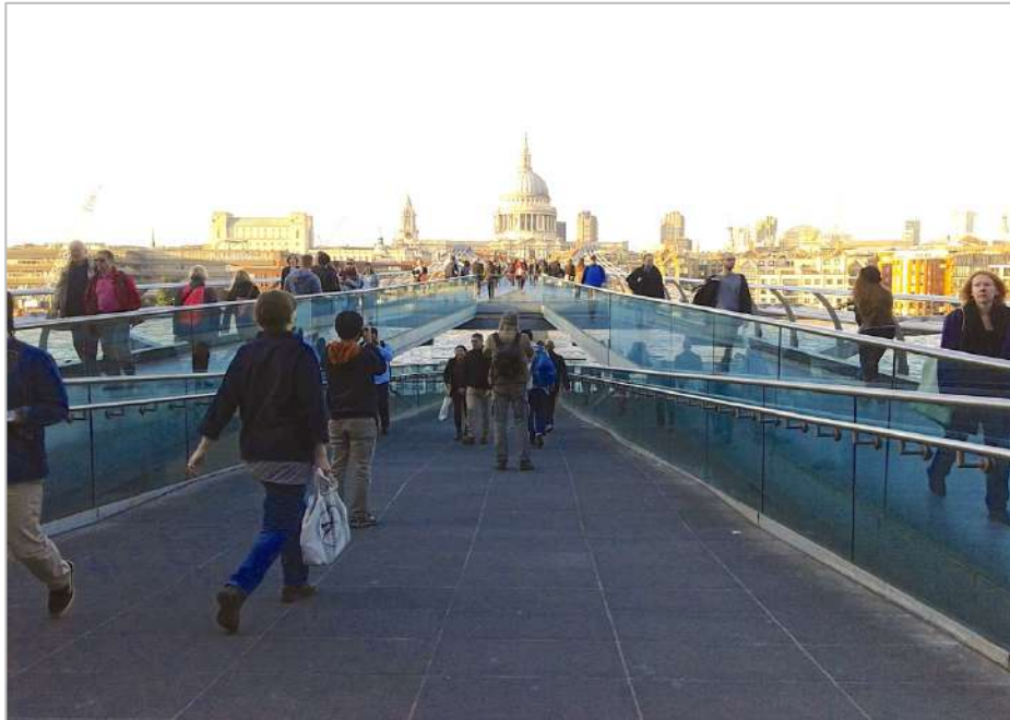
Millennium Bridge, London A footbridge designed to be used by everyone
