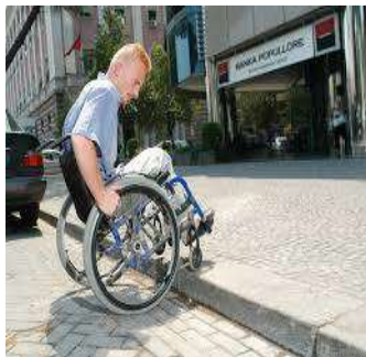
Lack of level access
